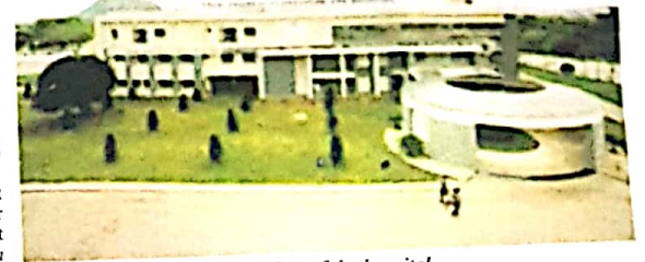
Front view of the hospital
